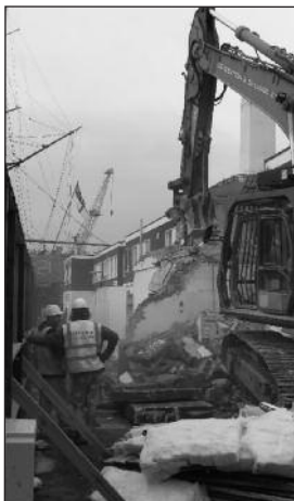
Demolition of Trafalgar Building.
